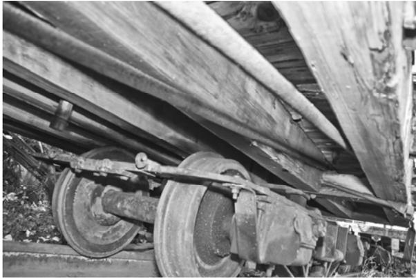
There are a number of places on both pages where the truck body bolster diagonal truss rod crosses from under the side sill of the car and angles upwards toward the intermediate sill and the centerline of the car. These photos and the top two on the next page are the winged truck with the extra hardware to hang the brakes from it. Compare the top bar of them to see the differences. Also look to see which is sprung.
